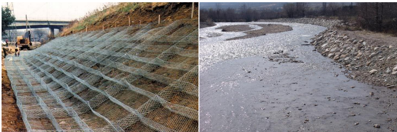
Figure 14. Bank Stabilization Solutions: Left: Model of a gabion mattress prepared to receive rockfalls (Arrigo Gabioni Inc); Right: the use of rockfalls for the protection of some banks
