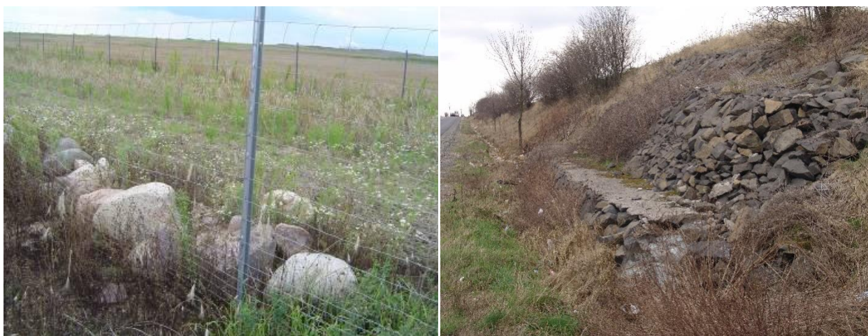
Figure 16. The use of microhabitats boulders that is able to provide additional environmental niches (left) and acting as a water drain zones of the washer which substantially contribute to stabilizing slopes (Right)
