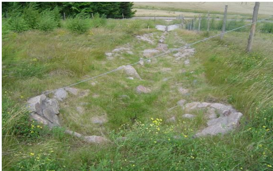
Figure 13. A model of a giant and reinforced stone gutter that ensures the drainage of rainwater in a manner that replicates natural structures
